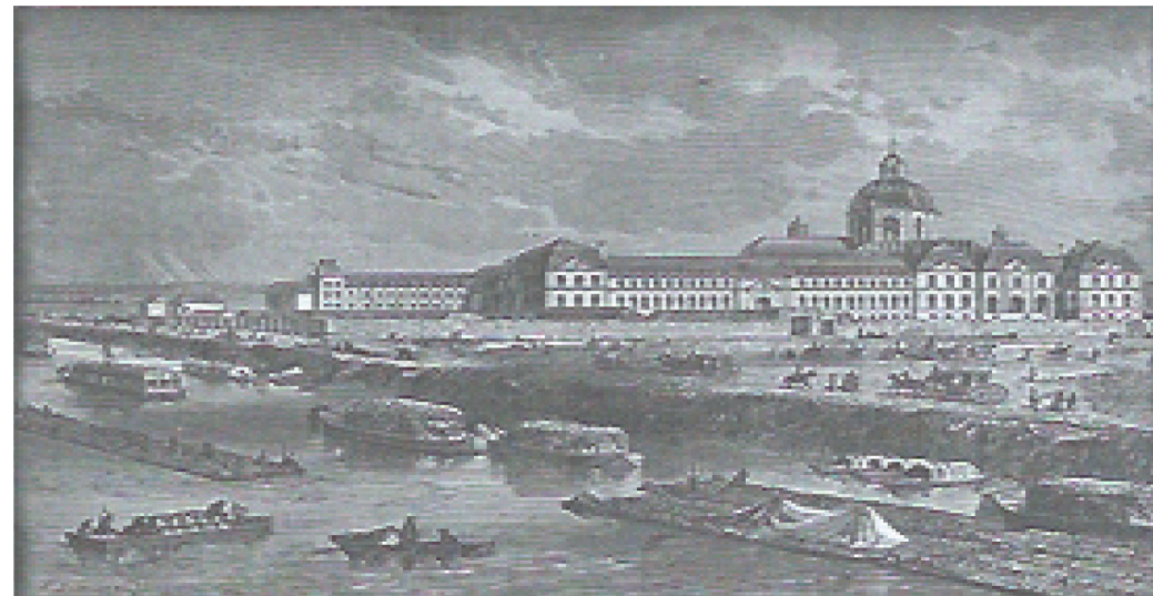
Figure n°3 – The General Hospital " Salpêtrière" is set back from the water way, for a long time the principal and founding activity of this site
